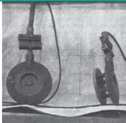
① Hopwood's directional hydrophone with baffle for submarine detection (1919).
